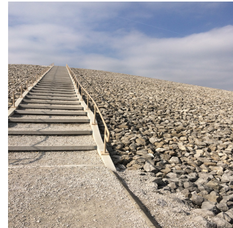
01 Weldon Spring disposal cell.
